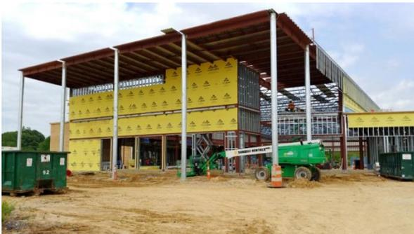
We are nevertheless making substantial progress, especially in 2019 with some drier weather. The concrete slab, with underlying data, electric, and water lines, is finished. The steel "skeleton" of the building is also done. The exterior walls are underway. We expect to have a "closing in" ceremony, with the building closed to the elements, in late August. We are still targeting a late 2019 opening. We hope you will join us!
